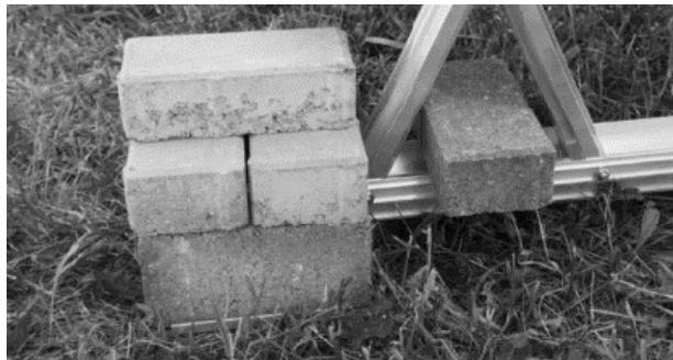
Apply ballasting according to the plan.
