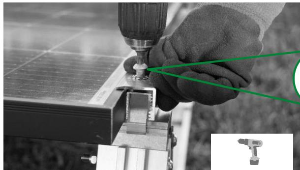
Tighten the screw while pressing down on the clamp
