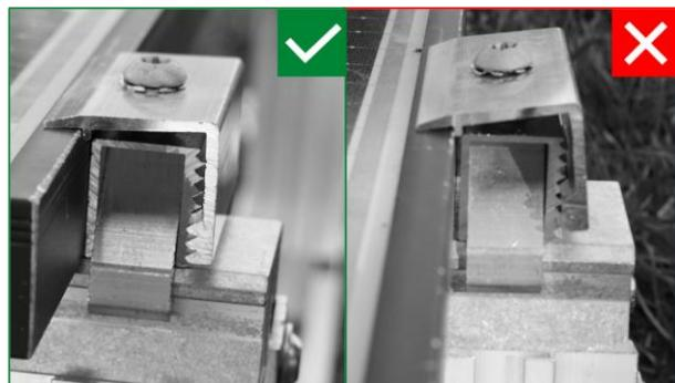
Before tightening: press down on the end clamp for the grooves to engage and the clamp to be in full contact with the module. Check if the fit is correct.
