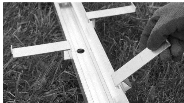
If required → Attach three ballast clips to the base set for subsequent ballasting with paving slabs. Arrange the clips as shown.
