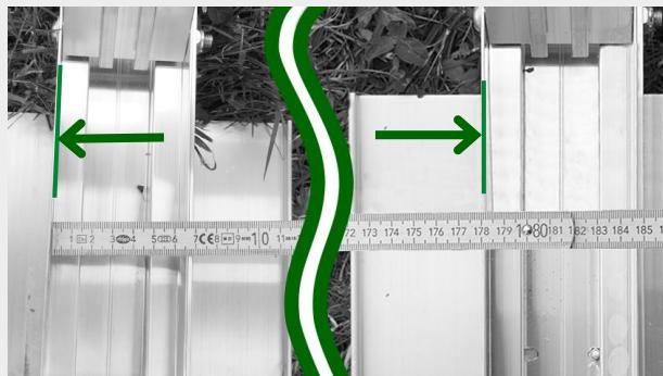
Place the tape measure at the left edge of one basic set and measure to the left edge of the next row.
