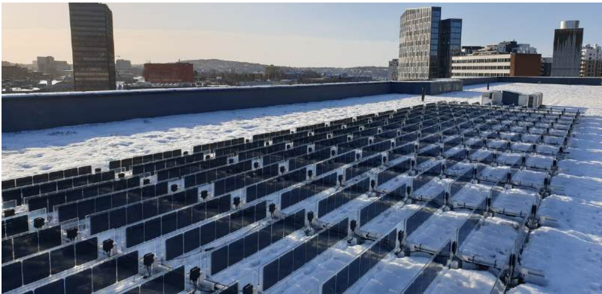
Vertical panels stay snow-free and benefit from high albedo
