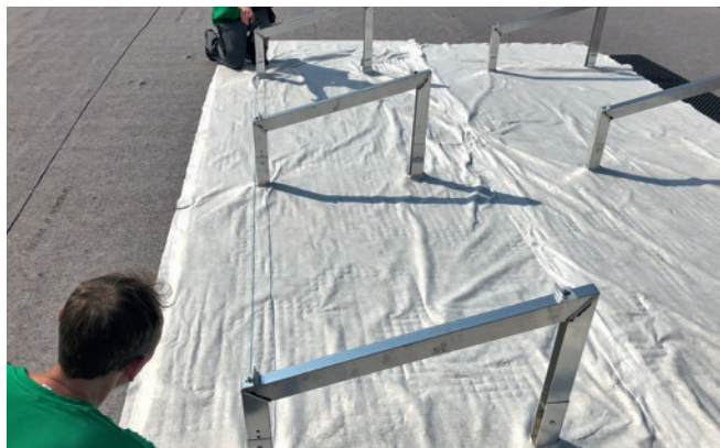
Figure 21: Alignment of the row using string
