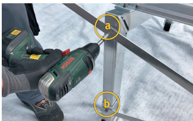
Figure 29: Position of drilled holes
