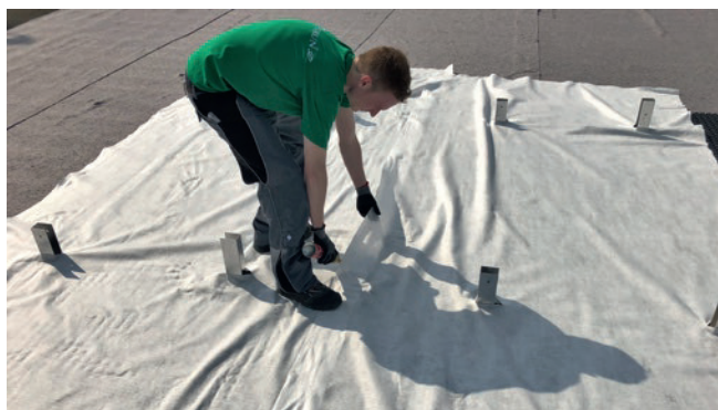
Figure 17: Bond rows of fleece with hand soldering iron
