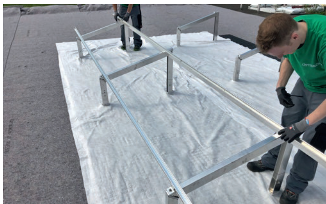
Figure 23: Mounting the second Easy Mounting Rail.
