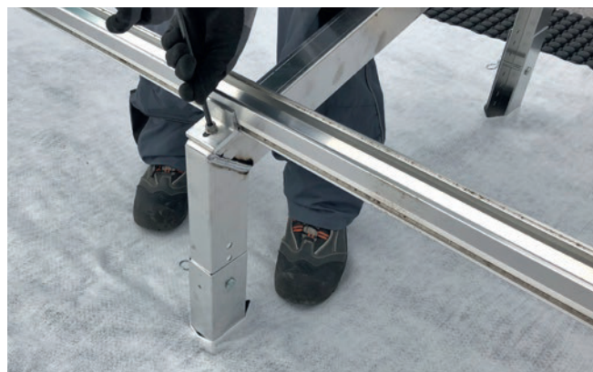
Figure 24: Tighten Rail Fixings.
