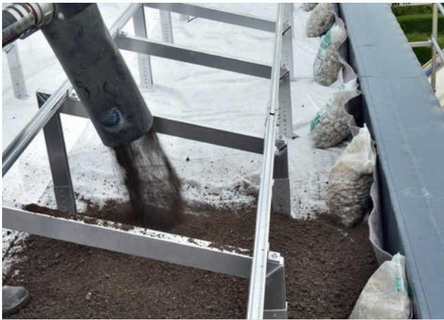
Figure 33: Blowing of the substrate.
