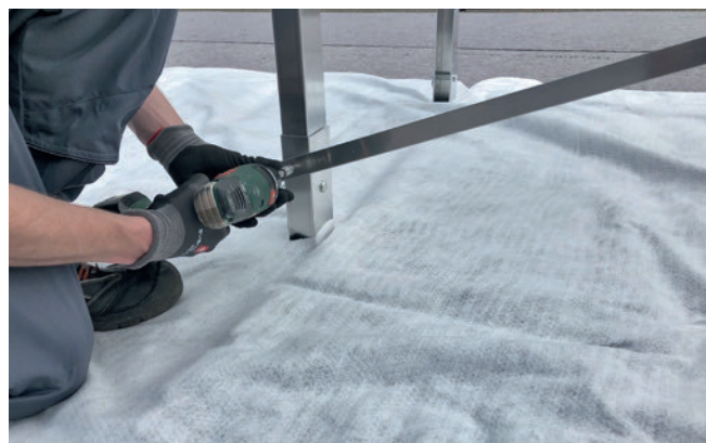
Figure 28: Fastening of the metal strip.
