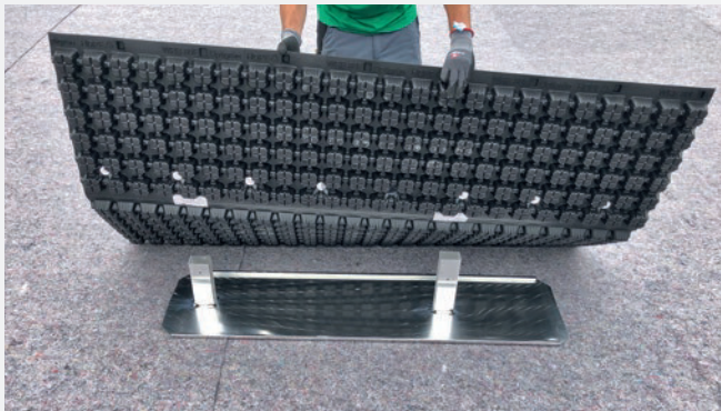
Figure 5: Laying out the Base Plate with WRB 8oFMA.
