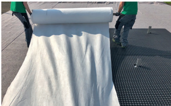
Figure 10: Rolling out the Filter Fleece.
