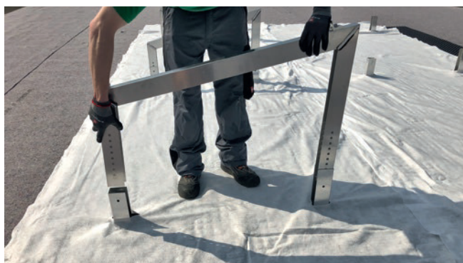
Figure 19: Mounting Frame on the Base Plate (example Mounting Frame).
