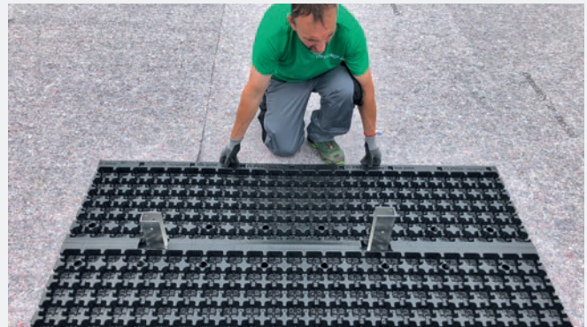
Figure 6: First WRB 8oFMA placed unfolded on Base Plate.
